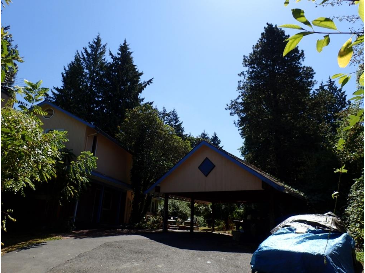
Photo 1: A view of some of the large coniferous trees and the two structures found onsite
